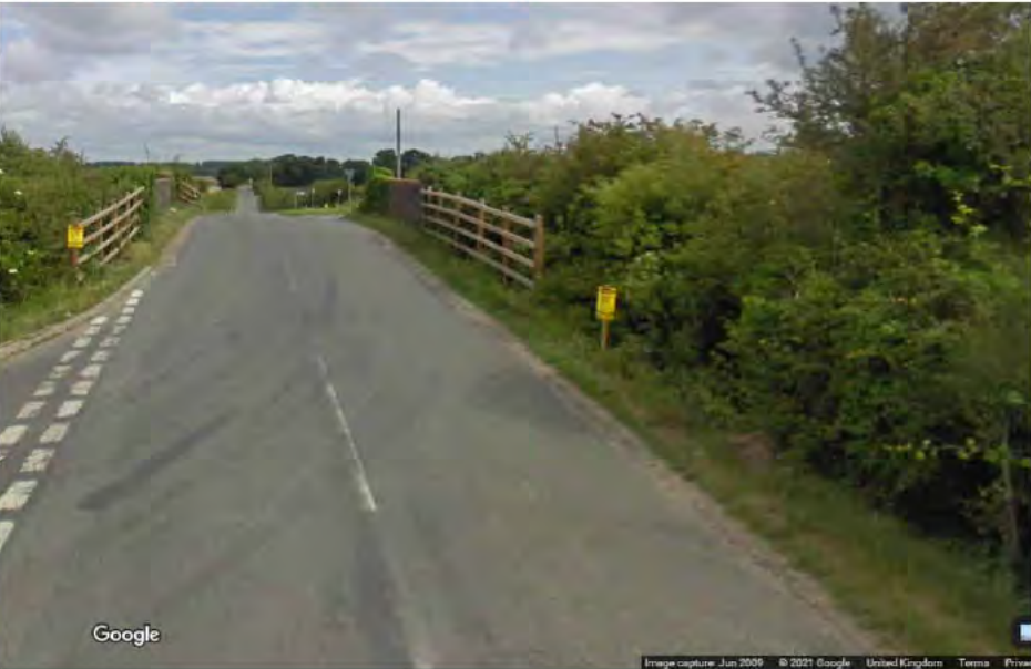
Figure 32: Google Street View of the Bridge
