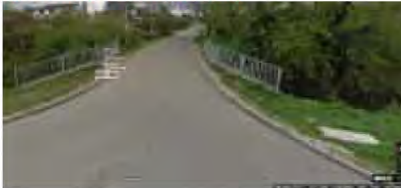
Figure 30: Google Street View Hythe Bridge
