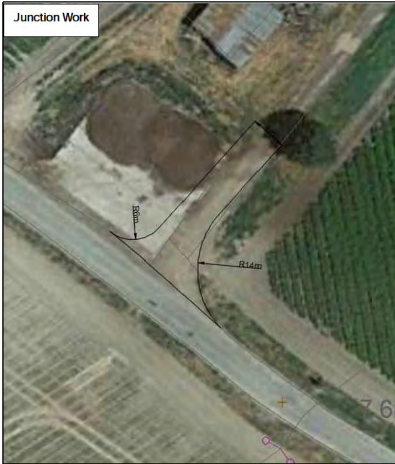
Figure 19: Sunnica East – Access F – Junction Work
